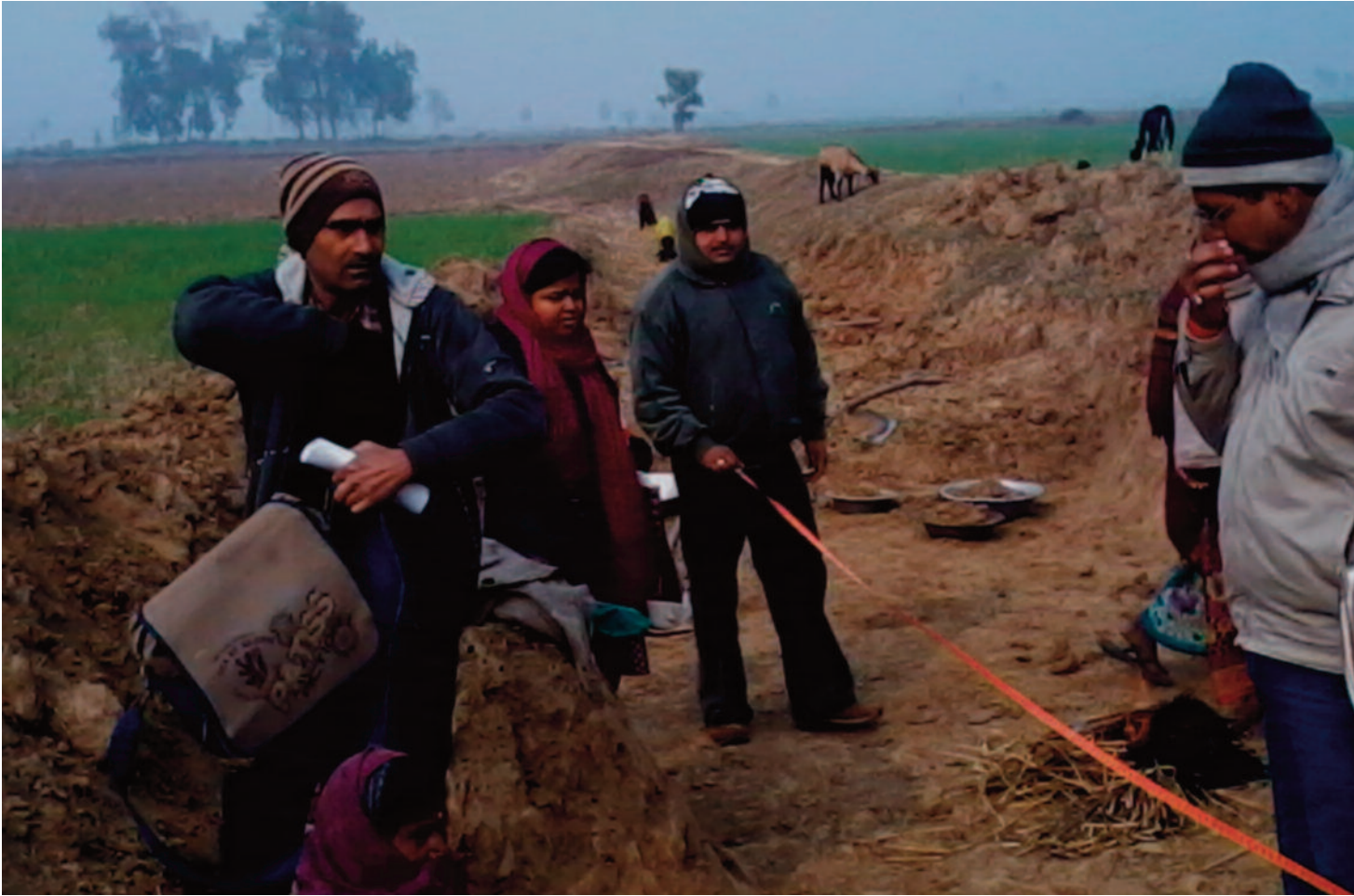
MGNREGA work in progress at Jehanabad
