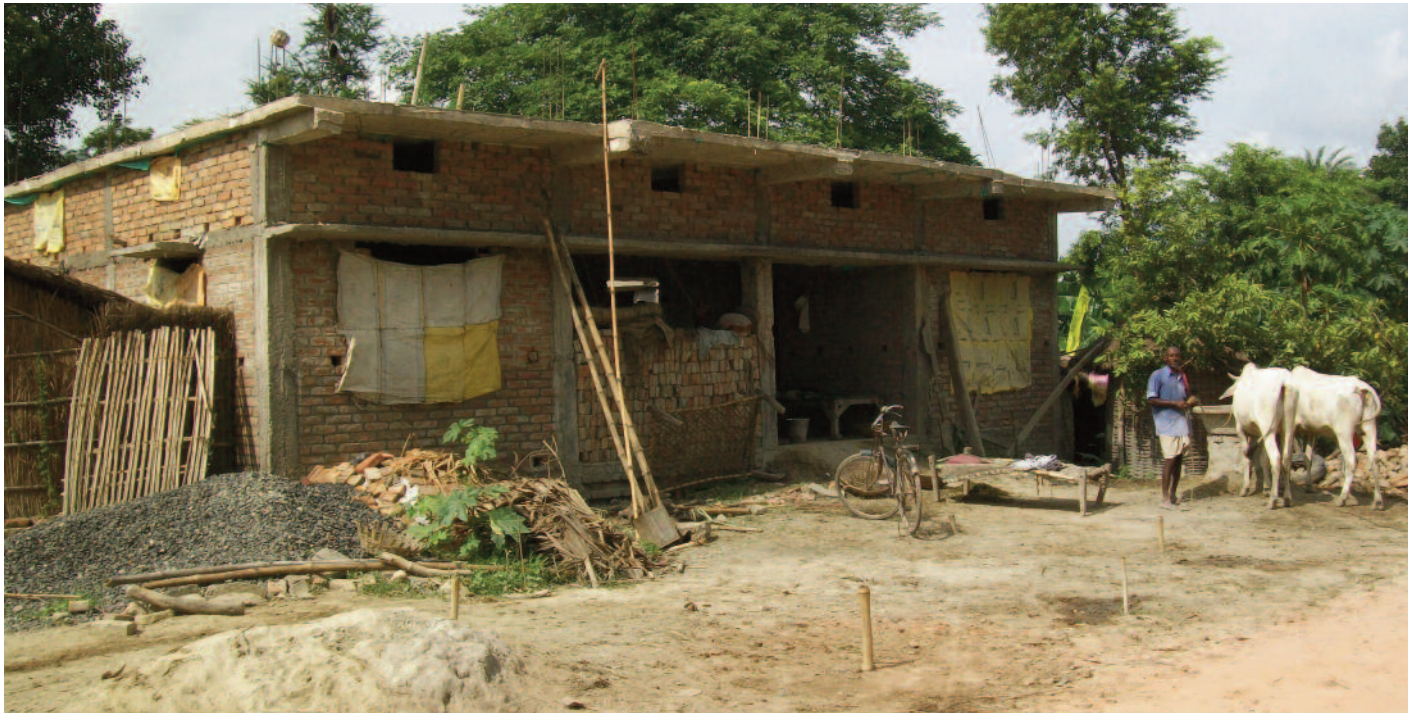
The under-construction houses, funded by Indira Awas Yojana, at Samastipur
