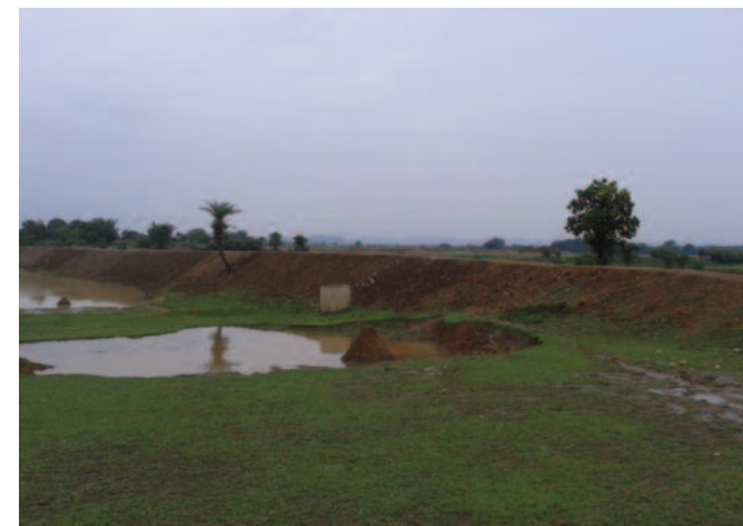
(From left) A newly built khet pokhari and MGNREGA workers at a construction site in the district
