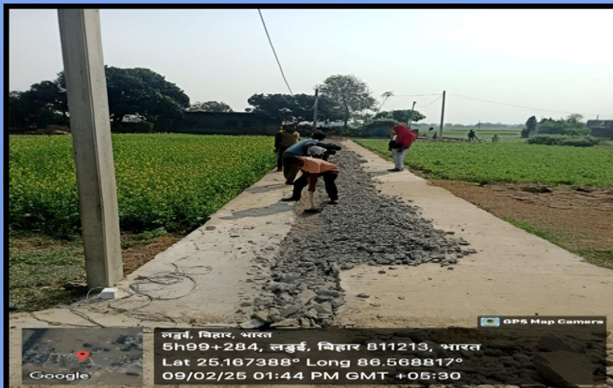
Restoration of P.C.C Roads and allied works
