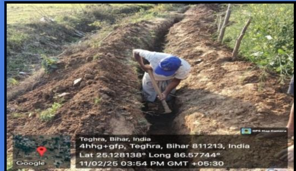
Laying of Pipe line:-Minimum Depth 1.1 M From G.L
