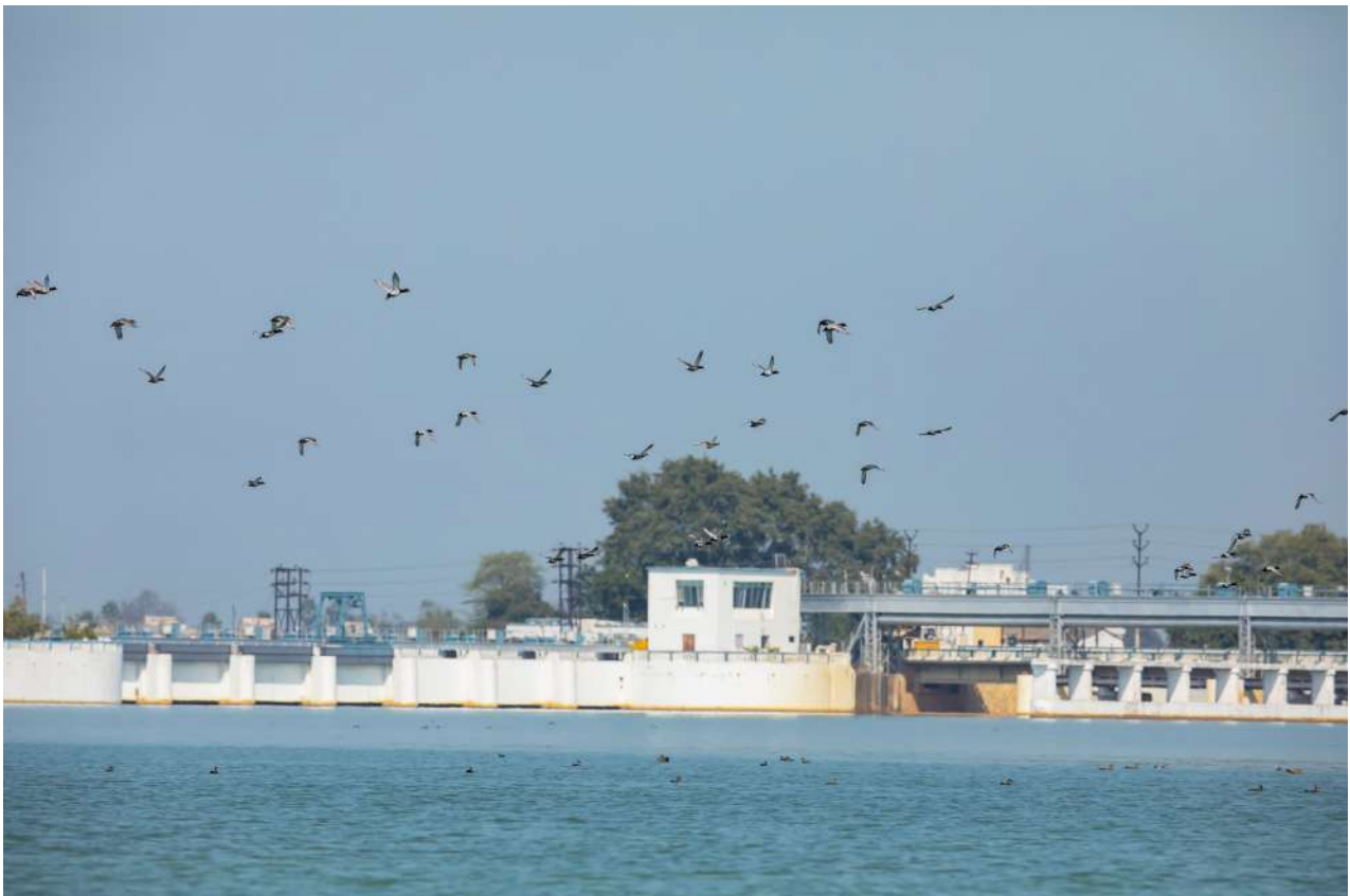
View of the Indrapuri Barrage
