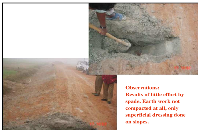
Photographs showing poor earth work in embankment
