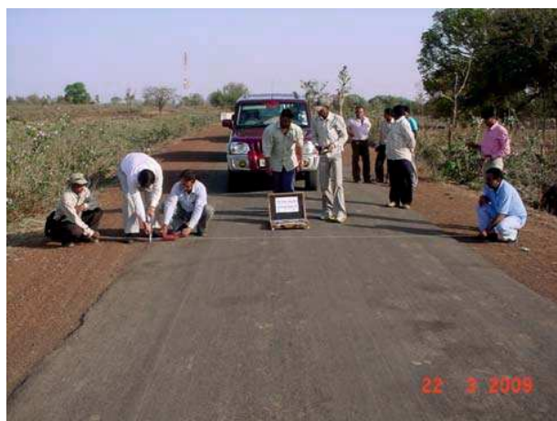
Photographs showing measurements of carriage way width, camber and super-elevation.
