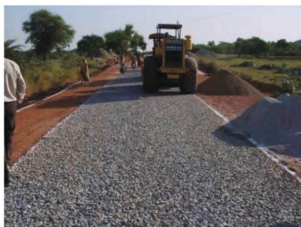
Photographs showing plastic GSB and good WBM work
