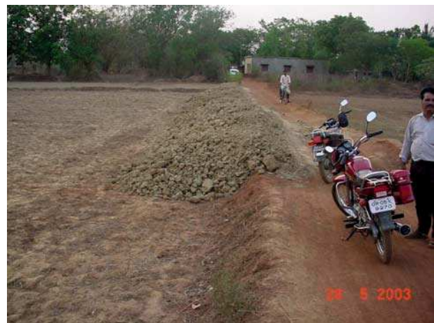
Photographs showing poor earth work in embankment
