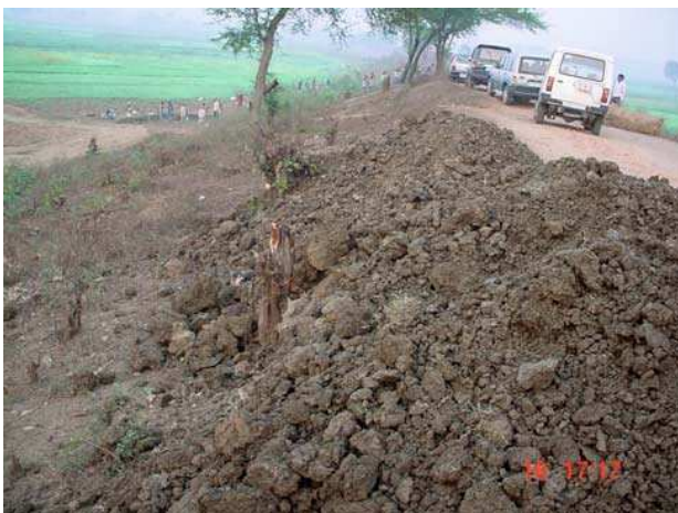
Photographs showing poor earth work in embankment
