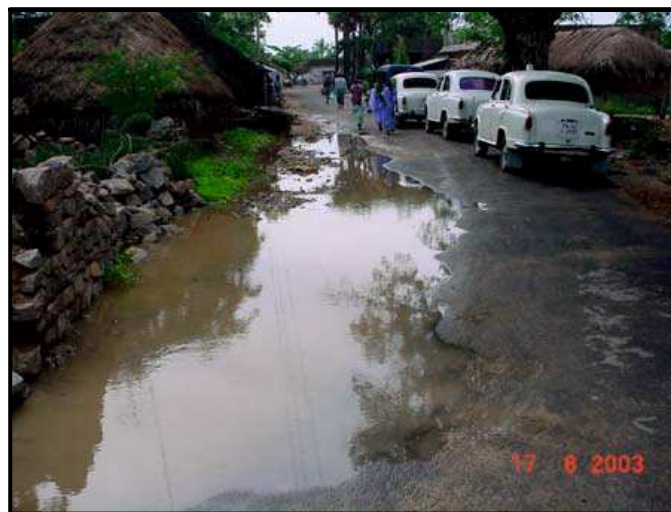
Photographs showing poor drainage.
