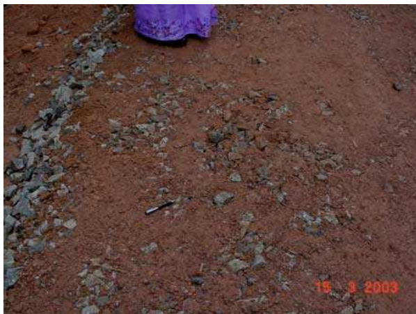
Photographs showing poor WBM and example of good WBM with good compaction
