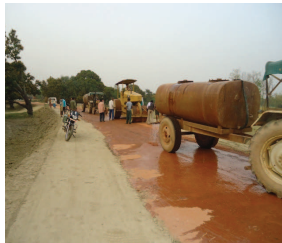
Photographs Showing WBM & Pre-mixing Work
