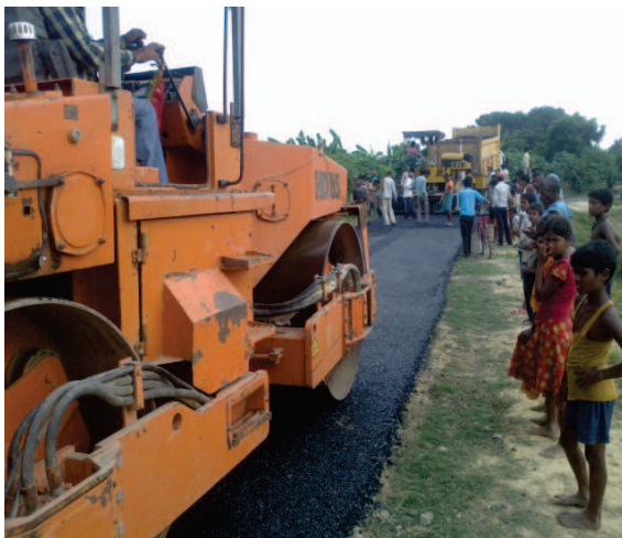
Photographs Showing WBM & Pre-mixing Work
