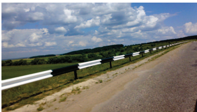
Photograph Showing Protection Work
