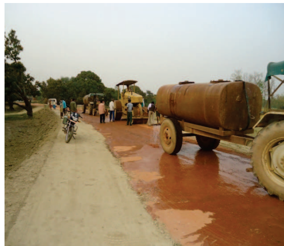
Photographs Showing WBM & Pre-mixing Work
